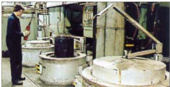
Convection type tempering furnace
