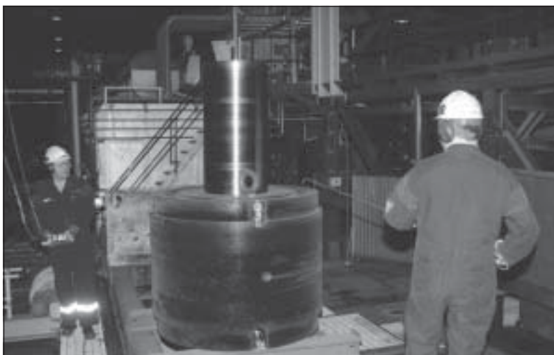
Shrinking of liner.
