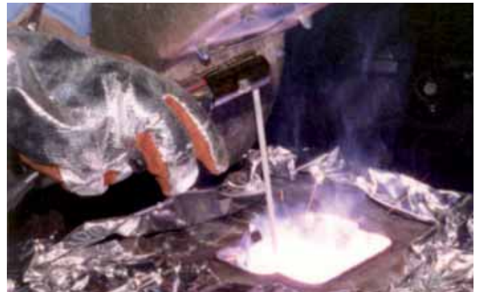
Manual arc welding and covering of components
