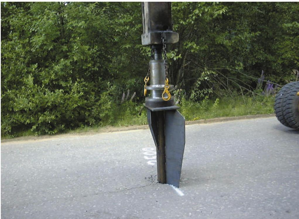
*Mandrel with attached welded footing for insertion into road asphalt as safety fence foundation.*
