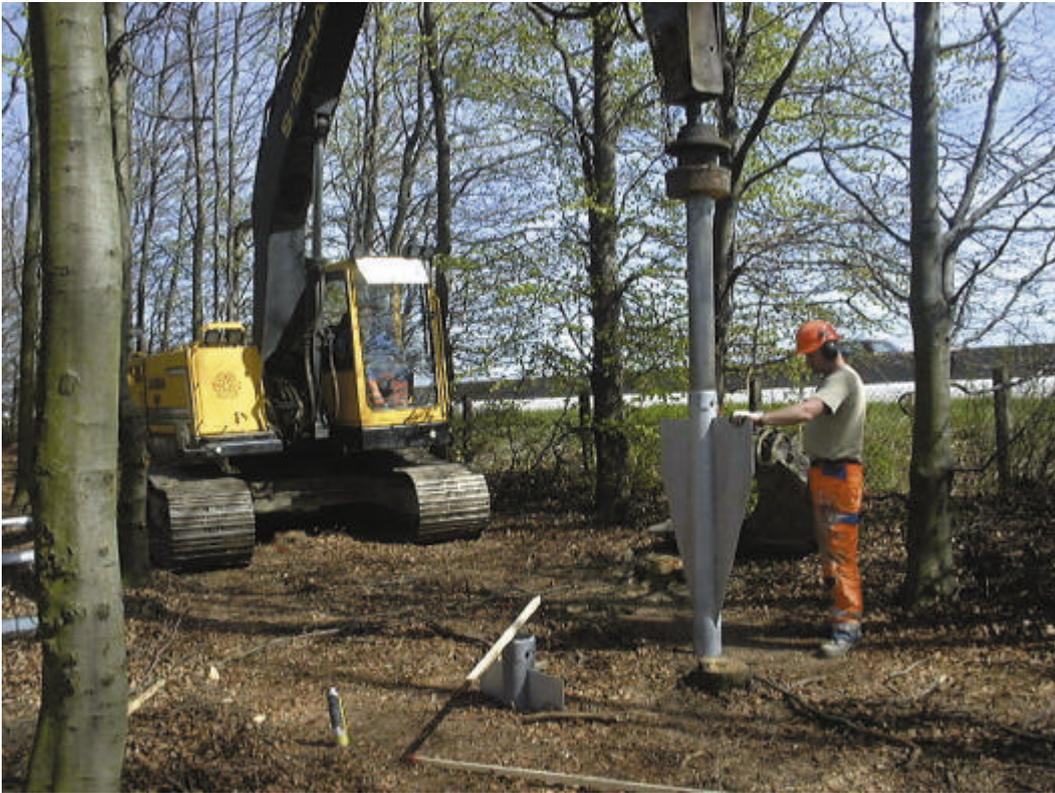
*Mandrel with attached welded footing for ground insertion of a foundation.*
