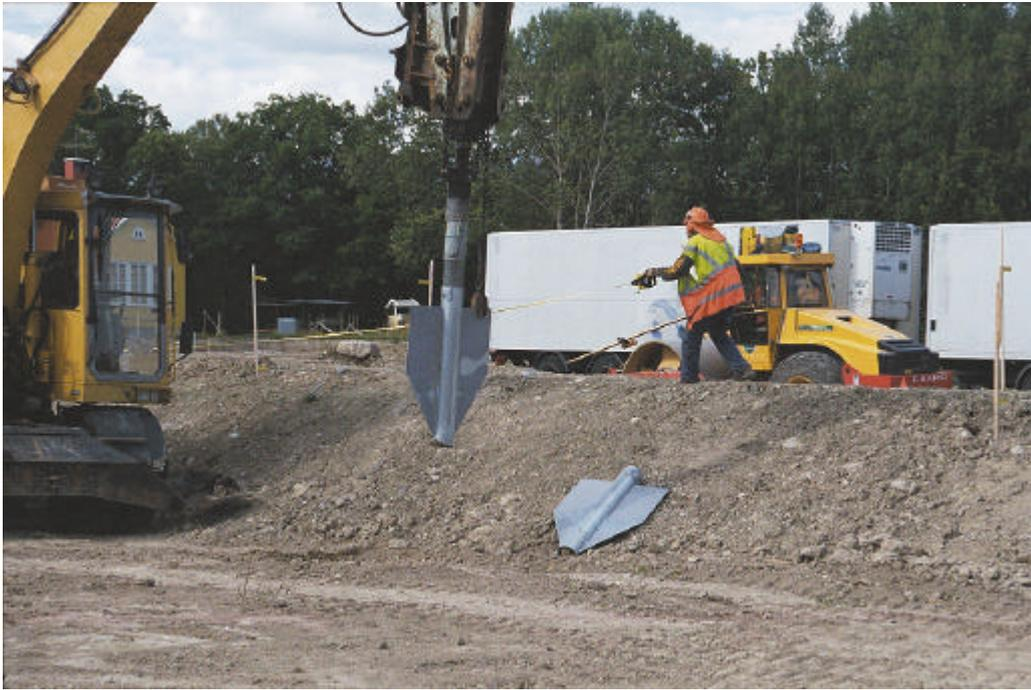
*Mandrel with attached welded footing for ground insertion of noise barrier foundation.*
